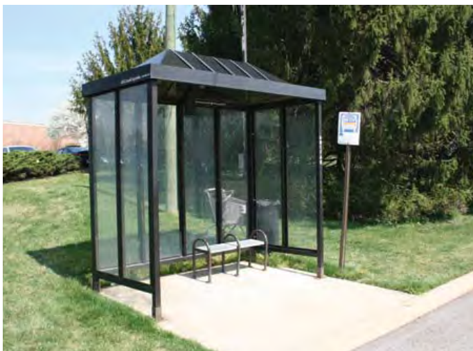
A bus shelter on Business Route 30, West Whiteland Township
