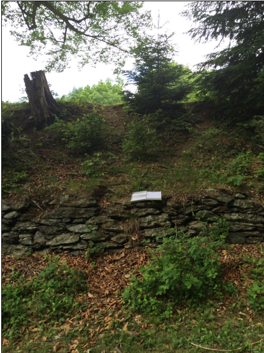
Photo 12. Downstream Face Northeast Side – Slope Erosion
