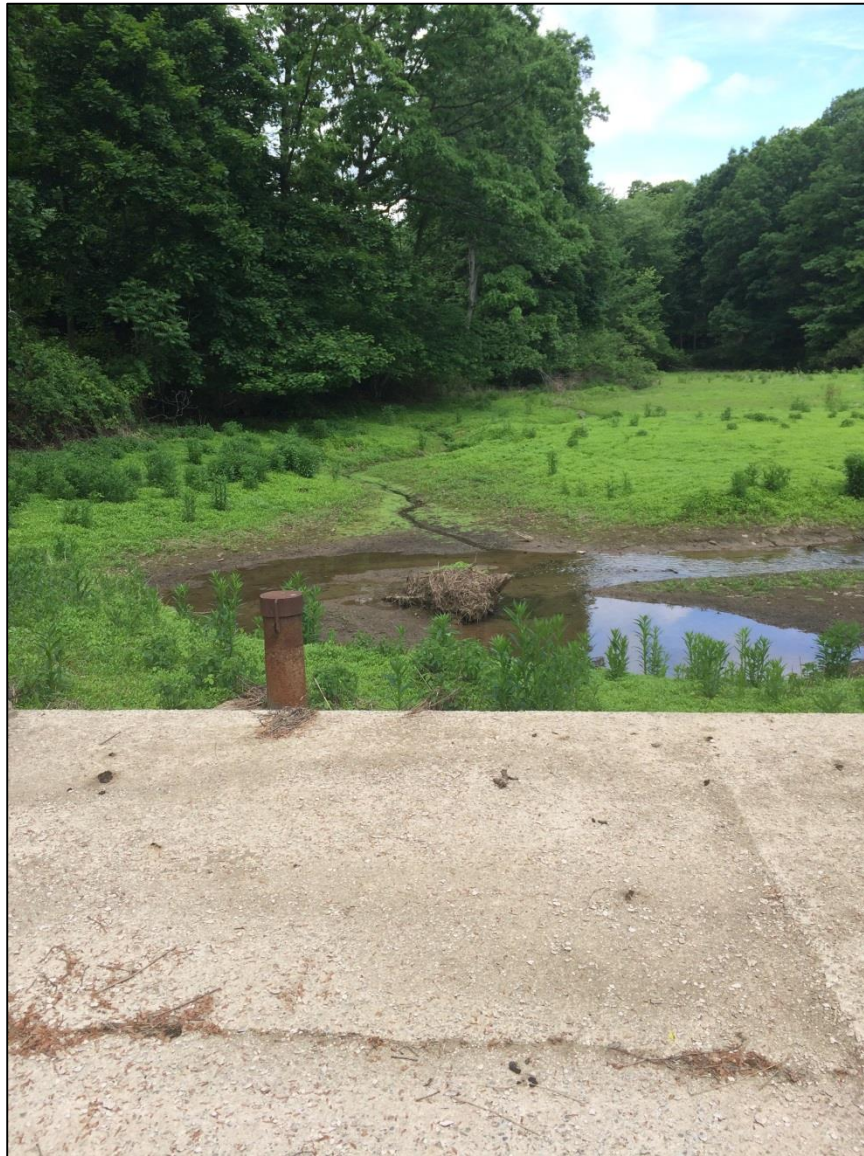
Photo 15. Outlet Control Valve Housing on Upstream Side of Spillway
