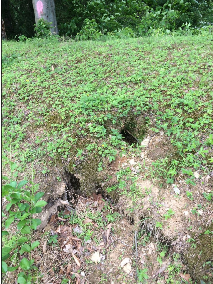
Photo 8. Upstream Face Northeast Side – Typical Void
