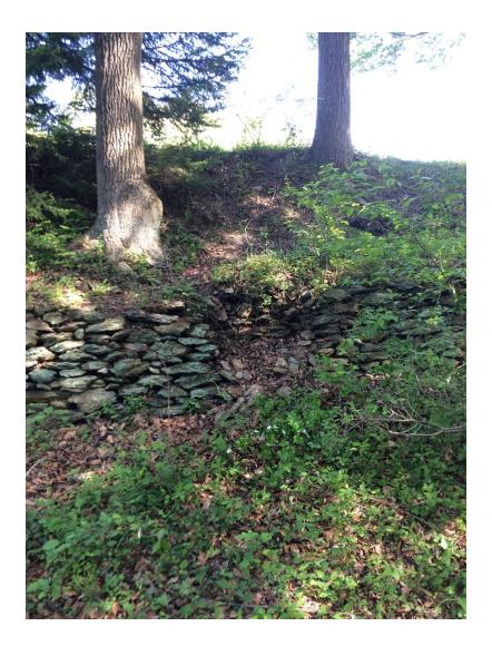
Photo 11. Downstream Face Northeast Side Looking North – Stone Wall in Disrepair
