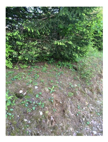
Photo 6. Typical Animal Burrows on Northeast Upstream Embankment Face
