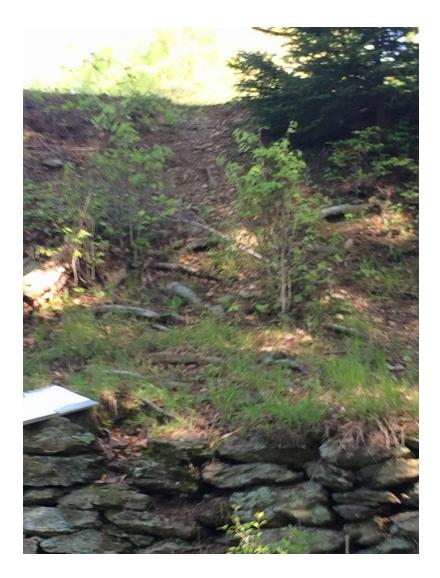
Photo 8. Downstream Face Northeast Side – Exposed Earth
