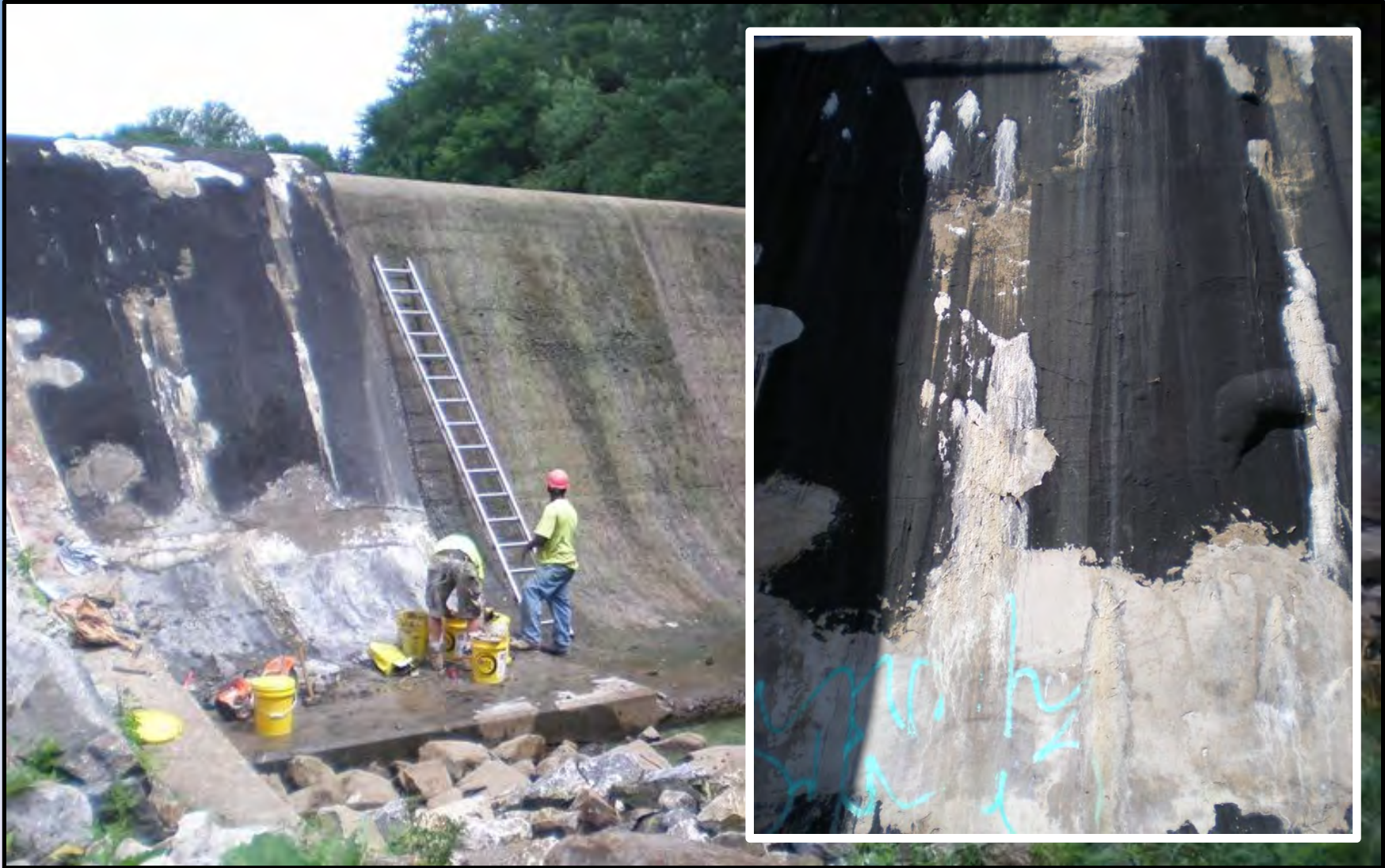
Application of liquid applied urethane coating to principal spillway surfaces. CIM 1000 Product by C.I.M. Industries, Inc.
