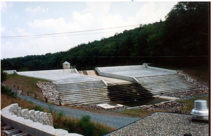
Figure 2-5: Long Run Dam No. 1 Repair. Gannett Fleming designed improvements to rehabilitate the Long Run Dam No. 1 to handle the full PMF.
