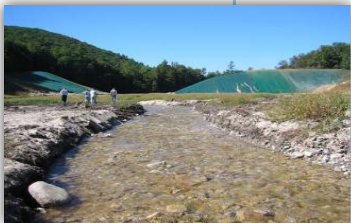
Figure 2-9: Birch Run Dam Evaluation and Breaching. After investigating alternatives, Gannett Fleming recommended breaching the Birch Run Dam due to safety concerns.
