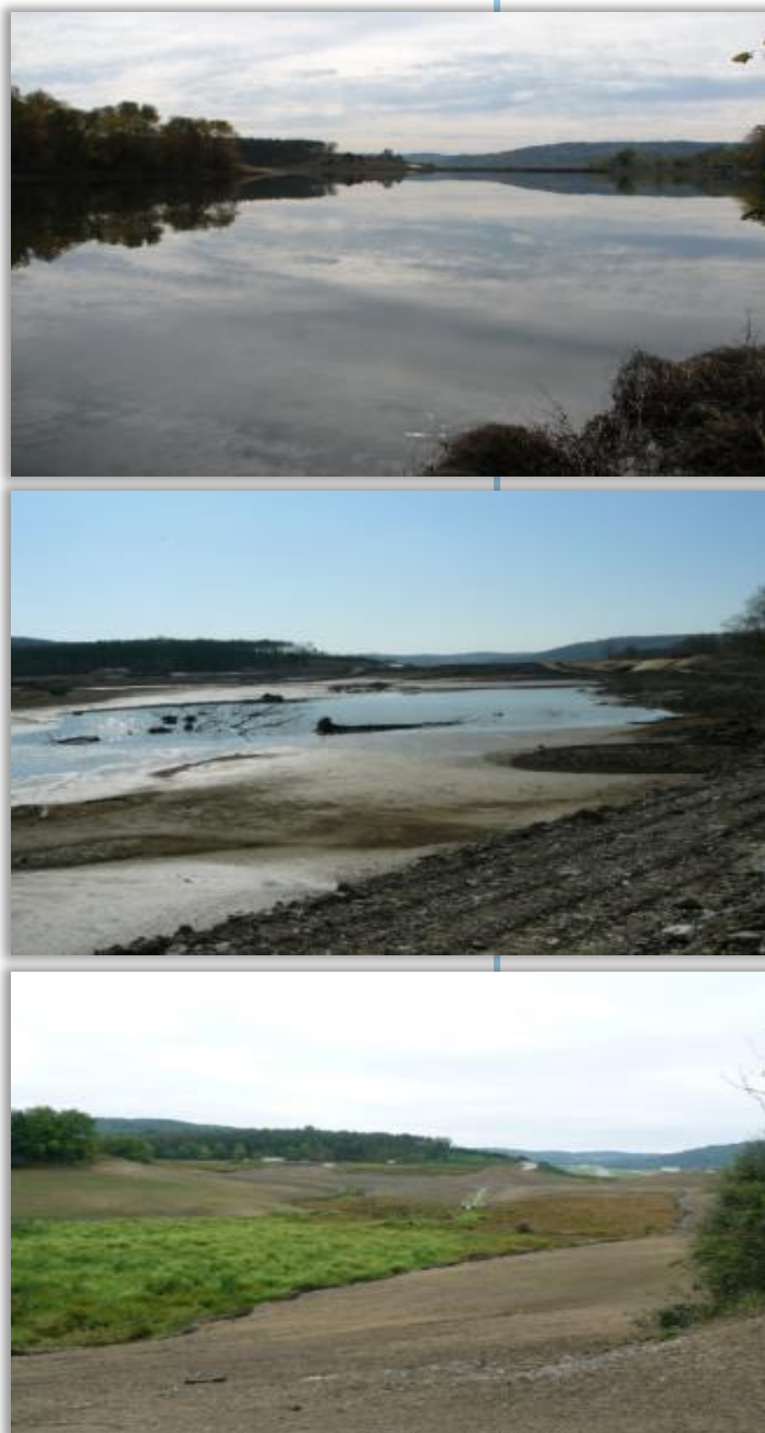
Figure 2-8: Breaching of Upper and Lower Hereford Manor Lake Dams. Due to safety concerns, Gannett Fleming prepared preliminary and final designs for breaching the dams, which is shown before, during, and after construction of a new box culvert under S.R. 588 immediately downstream of the lower dam.
