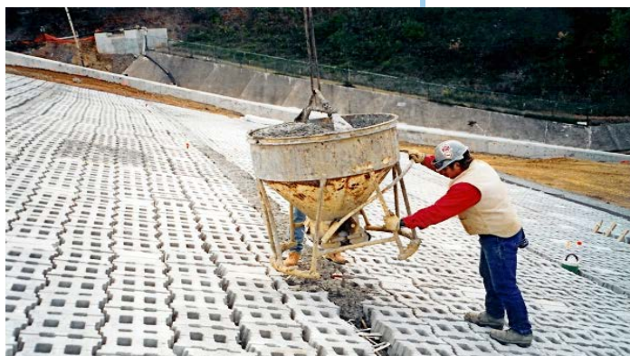
Figure 2-6: Shavers Creek Dam Repair. Gannett Fleming designed improvements to eliminate voids under the spillway and improve the dam to meet PADEP requirements.
