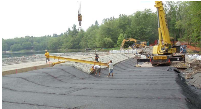
Figure 2: Articulating Concrete Block (ACB) Placement at Lake Natalie Dam. ACB is one option for overtopping protection that could be considered for Milltown Dam.
