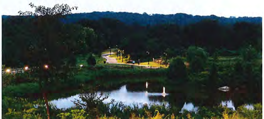
Wilson Farm Park, Tredyffrin Township, Chester County, PA . Here SC create a 2-acre water feature that is the park's storm-water management basin and the source of irrigation for the parks 7 sports fields. This has been in operation for over 10 years.
