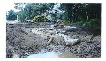
should be high marsh (up to 6" deep) and half should be low marsh (6" to 18" deep). Varying depths throughout the CWs can improve plant diversity and health. The open water zone (approx. 35 to 40% of the total surface area) should be between 18 inches and 6 feet deep. Allowing a limited 5-foot deep area can prevent short-circuiting by encouraging mixing, enhance aeration of water, prevent resuspension, minimize thermal
