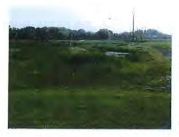
Constructed Wetlands are shallow marsh systems planted with emergent vegetation that are designed to treat stormwater runoff.
