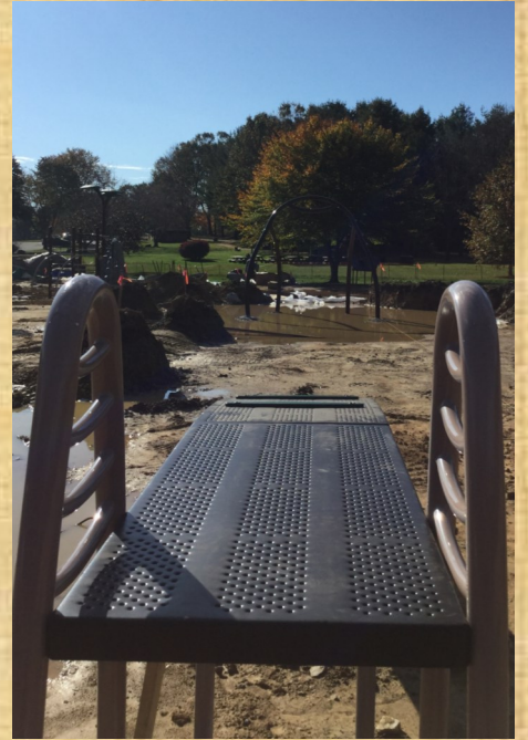
View from the 75' zip line launch deck
