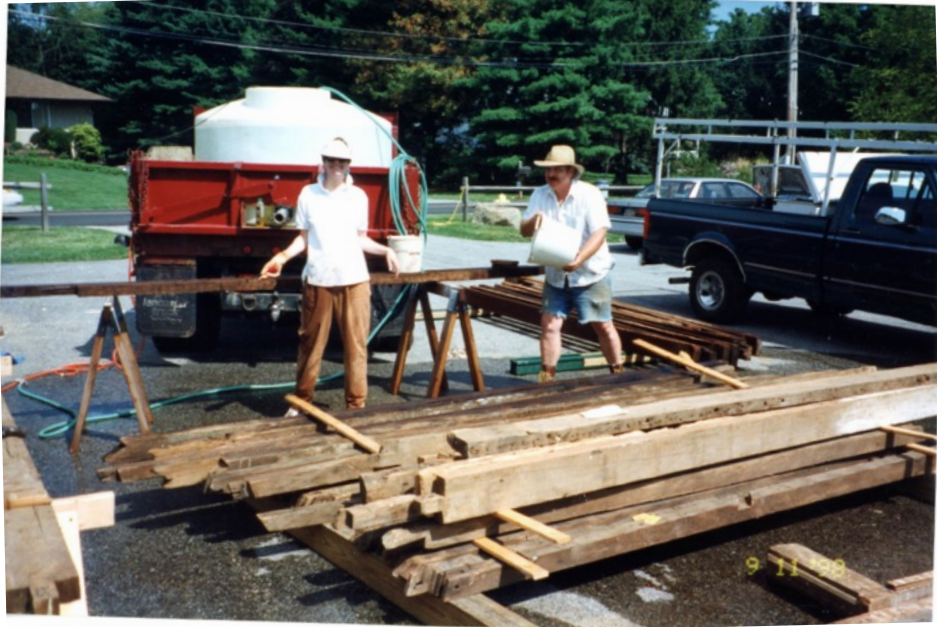
Washing of Planks prior to placement
