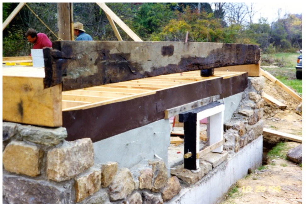
New Foundation with first planks
