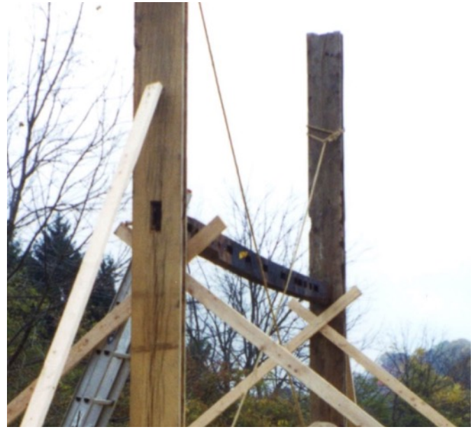
Center Posts in place
