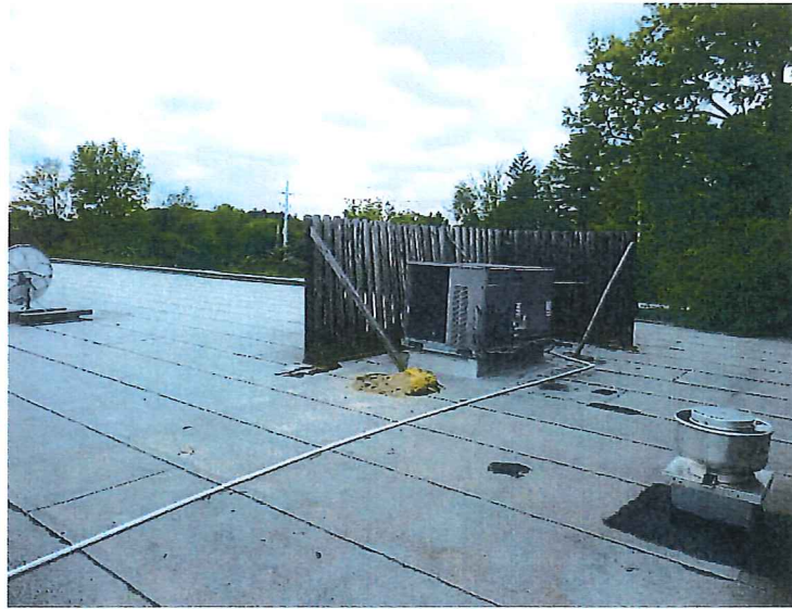
Roofing Photo R 3: Mechanical unit and screening
