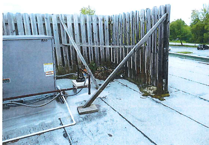
Roofing Photo R 4: Vegetation growing at screen base
