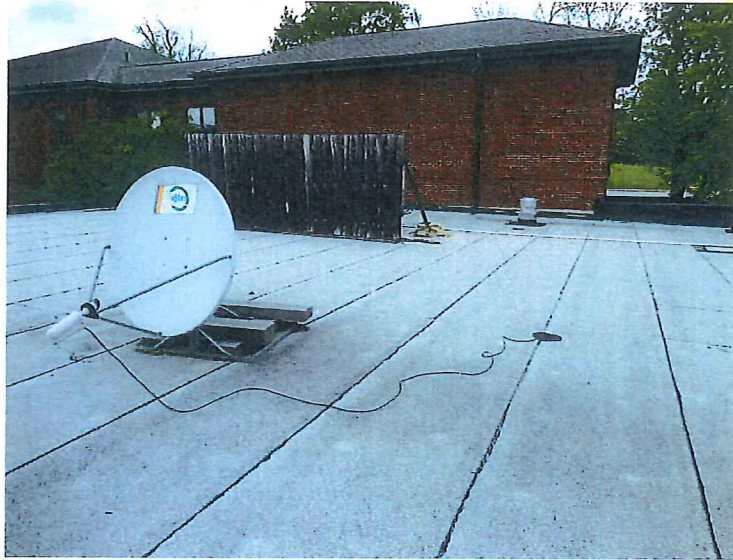
Roofing Photo R 7: Satellite dish on sled with ballast
