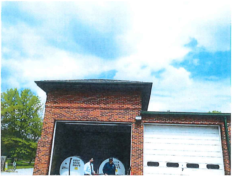
Roofing Photo R 2: Garage
