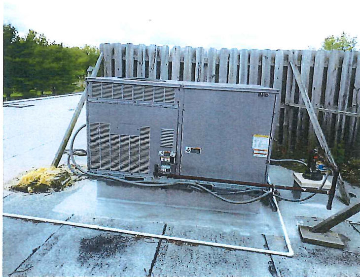
Roofing Photo R 5: PVC pipe installed at condensate
