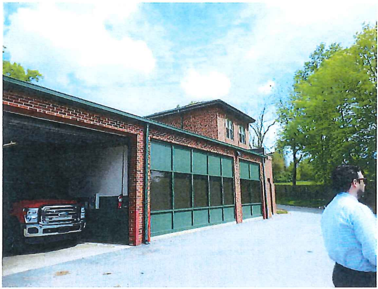
Roofing Photo R 1: Garage and Municipal Building
