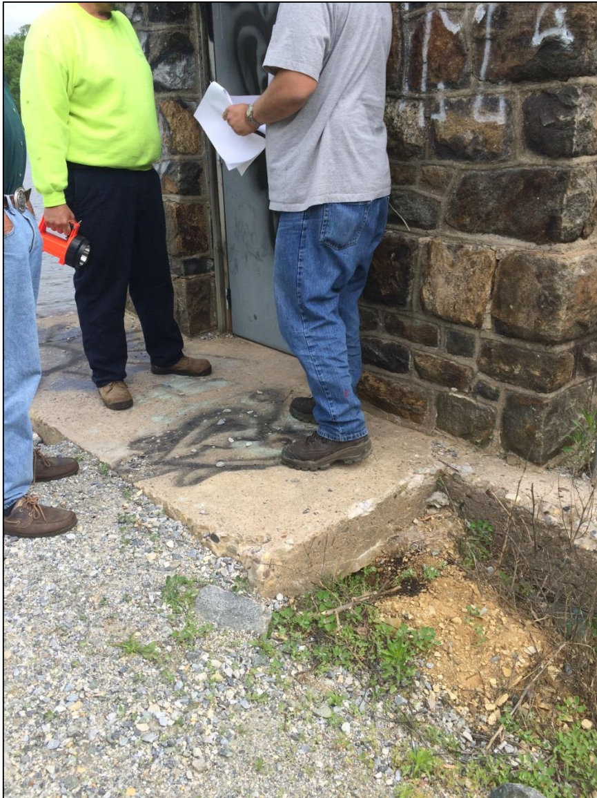
Photo 12. Outlet void facing downstream
