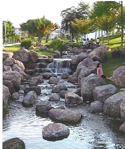
Constructed stream step pools can be used to prevent stream head cutting after a dam removal.
