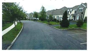
The general cartway width (curb to curb) of each roadway is 25 feet. Neither roadway is posted for 'No Parking', meaning parking 'on street' is allowed. Each housing unit has a two-vehicle garage along with some driveway parking capabilities. Also notable are the numerous three to five space parking bays along both roadways within the community. Those spaces are to provide for short term guest parking to the residences.
