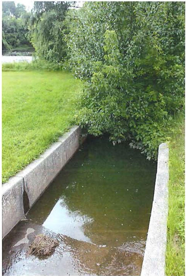
The channel which connects the pond and basin has been damaged by overgrown vegetation, which causes water to stop, stagnate and grow algae.
