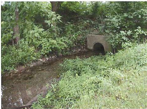
The existing channel entering the pond could potentially be converted into a forebay, to capture sediment in a smaller area before it enters the pond.
