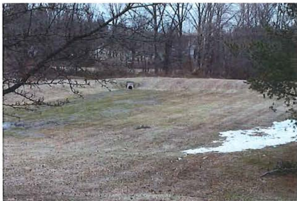
Over the past few decades, it's been determined that conventional basins are ineffective in managing stormwater, leading to degradation of area streams.
