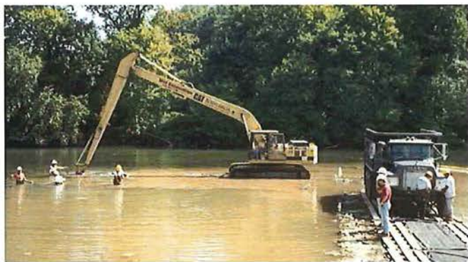
Dredging may be necessary at some of the ponds, as they have filled with sediment. CREDIT: Toth Brothers Clearing and Dredging
