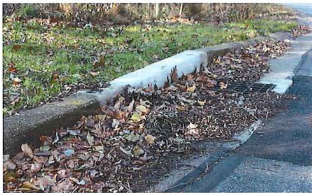
Inlets feed stormwater, and sediment and pollutants, from the streets into the ponds.
