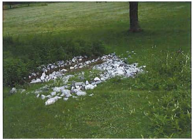
The existing spillway is unstable, and should be reconstructed. Additional plantings could also help to stabilize the banks.
