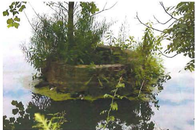
A sycamore tree is growing out of the outflow structure at Marydell and should be removed.
