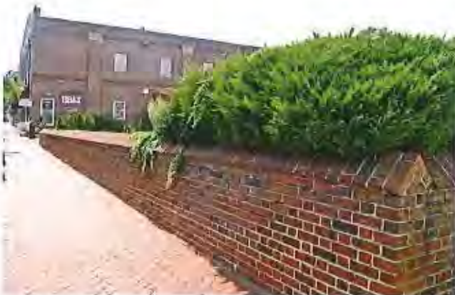
Brick Wall screening off-street parking
