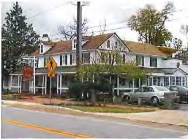
Off-street Parking located to the side of the building
