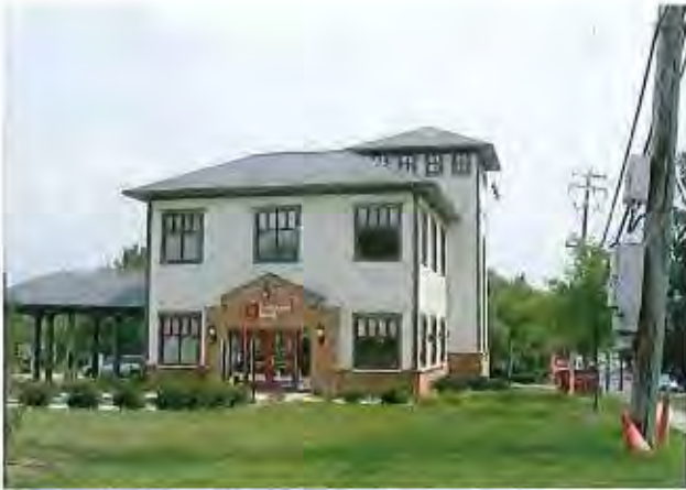
Bank with Drive-Thru Facility located in the rear
