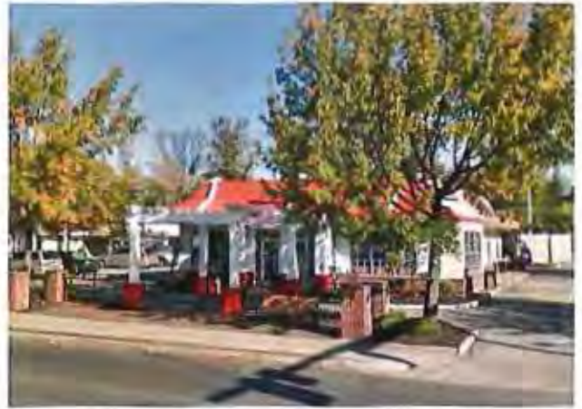
Existing Building with Pergola as transitional feature
