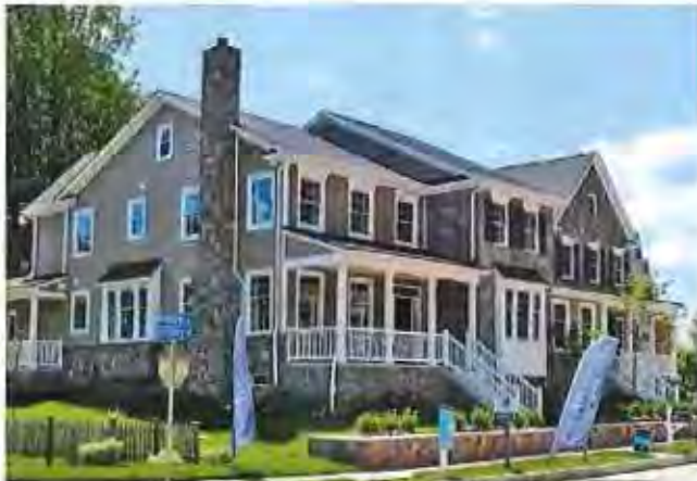
Building recesses and projections
