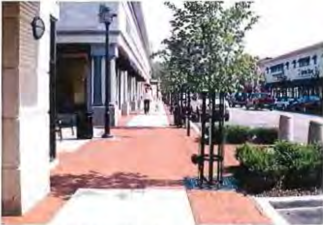
Buildings adjoining sidewalk
