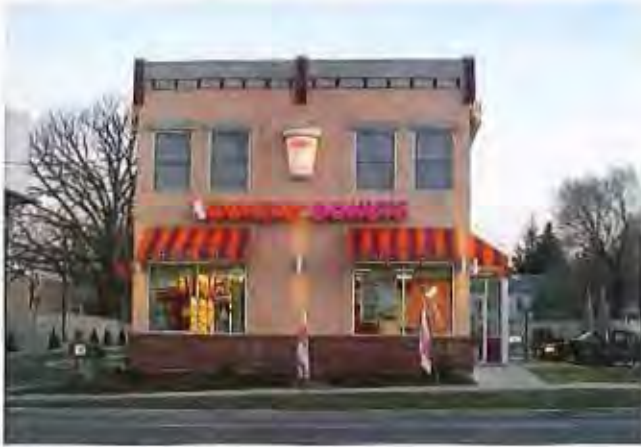
Building located at Build-To-Line.
