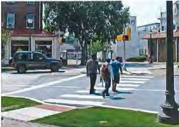
Crosswalk Striping connecting opposing accessible sidewalk ramps
