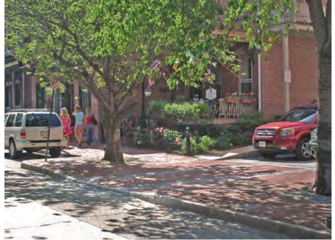
Curb Cut allowing continuous Pedestrian access
