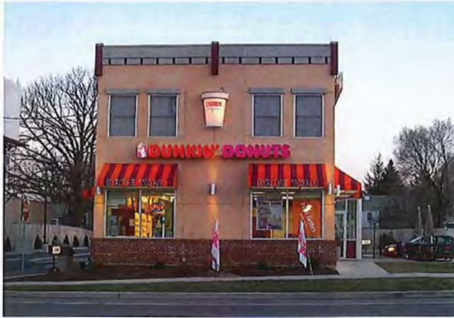
Building located at Build-To-Line
