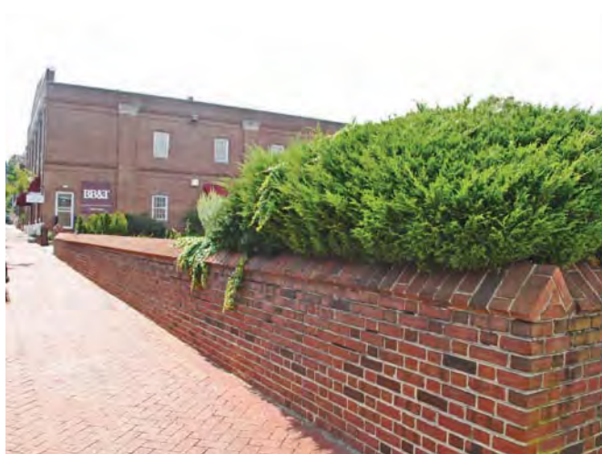
Brick Wall screening off-street parking
