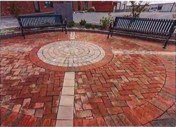
Brick utilized in Pedestrian Gathering Area
