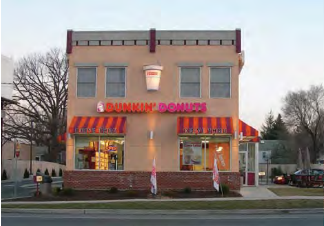
Building located at Build-To-Line
