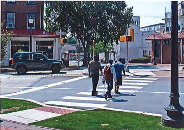
Crosswalk Striping connecting opposing accessible sidewalk ramps
