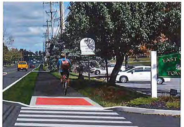
Multi-Use Trail and Crosswalk along Paoli Pike
