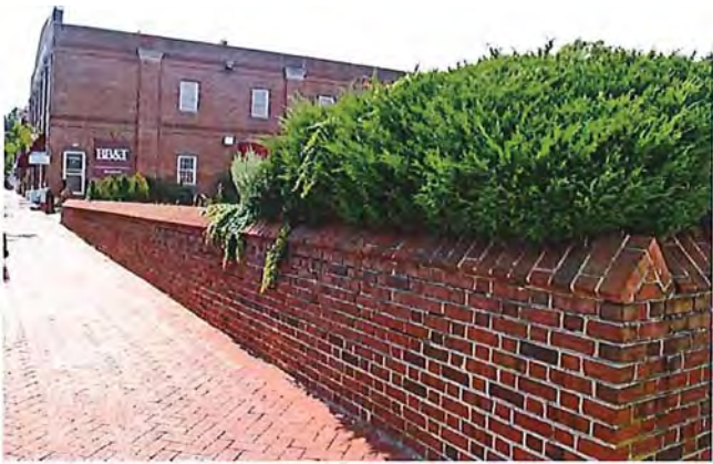
Brick Wall screening off-street parking
