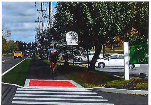
Multi-Use Trail and Crosswalk along Paoli Pike
