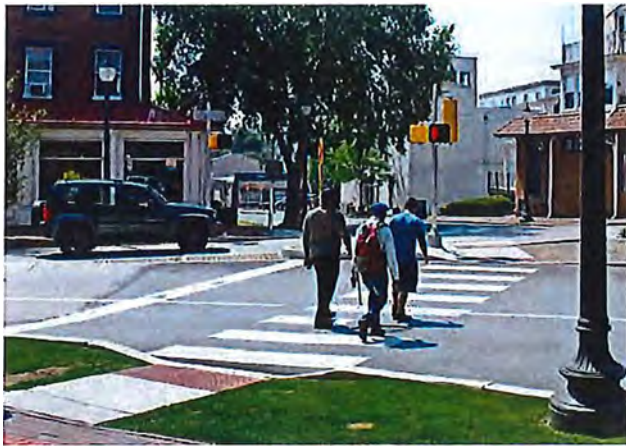
Crosswalk Striping connecting opposing accessible sidewalk ramps
