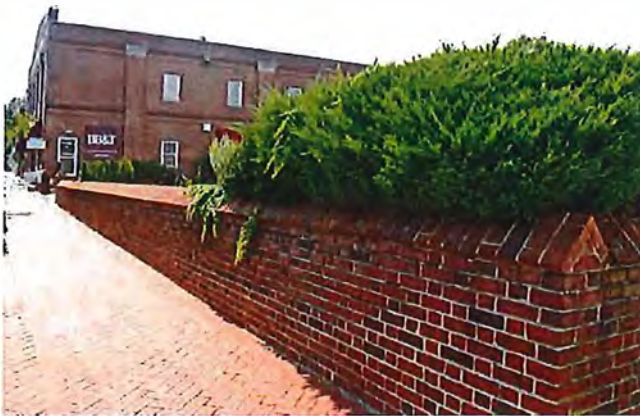
Brick Wall screening off-street parking
