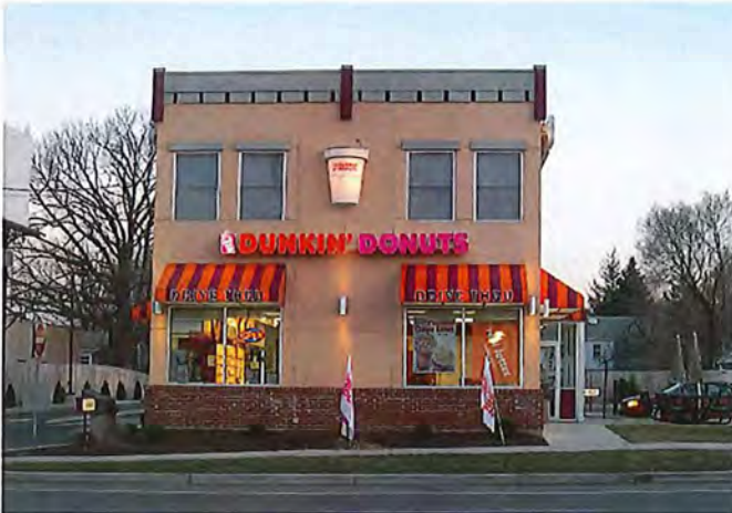
Building located at minimum front yard setback
