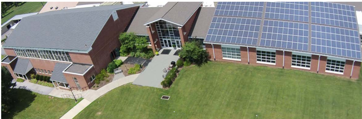
Solar PV on Westtown School Athletic Center
