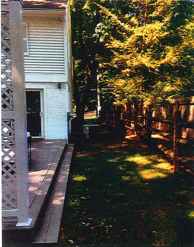
West view showing north property line and non-conforming structure and deck (property line is between the fences)
