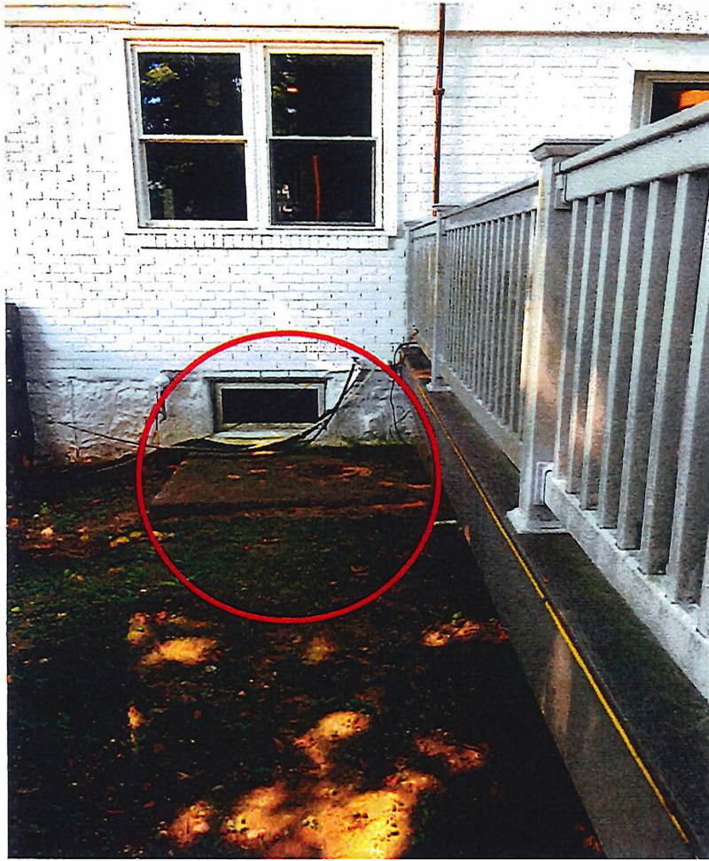
View of southern end of east elevation
