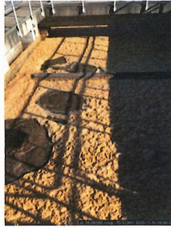
Description: SBR 4 Aerated fill
