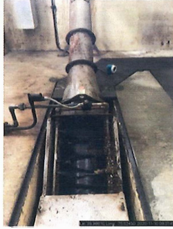
Description: Mechanical screen
