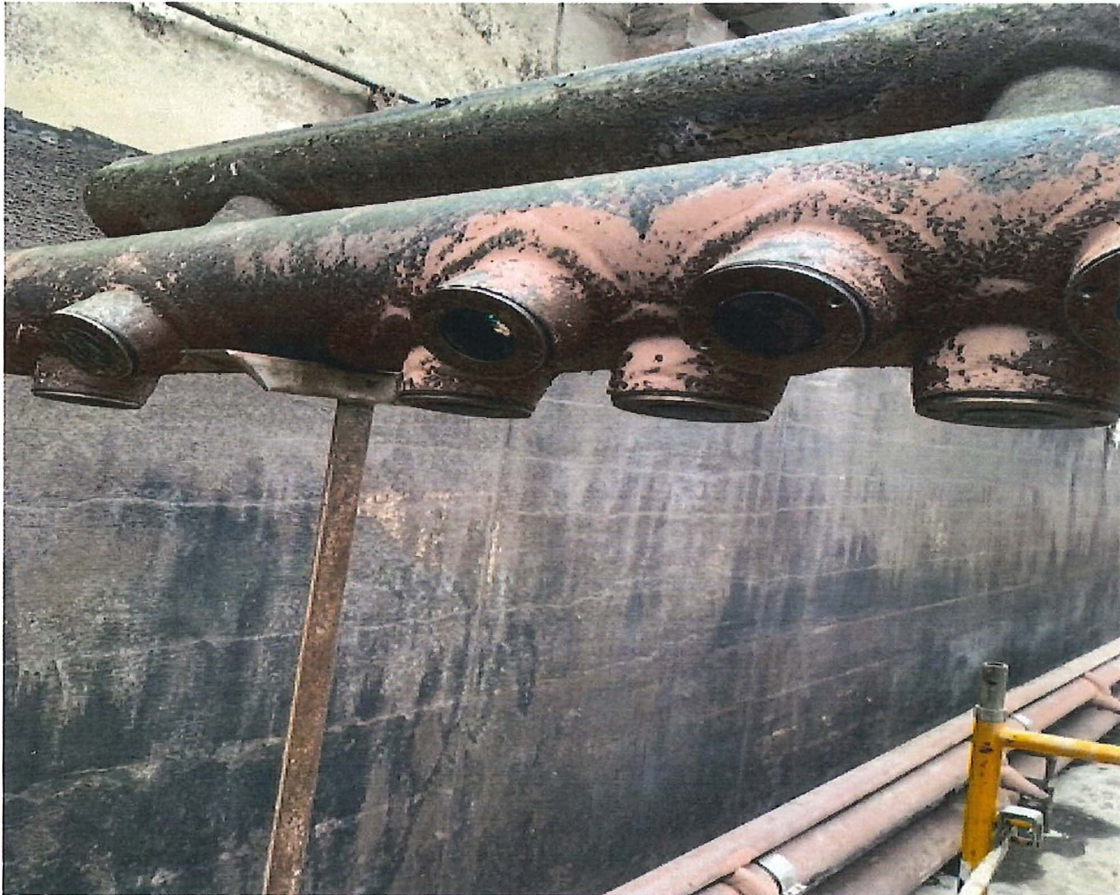
Figure 1SBR 4 decant Valves
