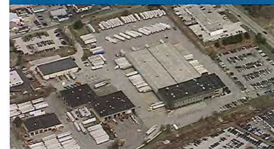
Light industrial/warehouse (located in areas that are separated from community-centric uses)
