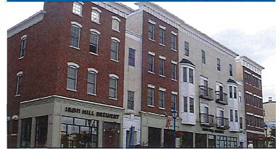
Ground floor commercial space in multi-story buildings
