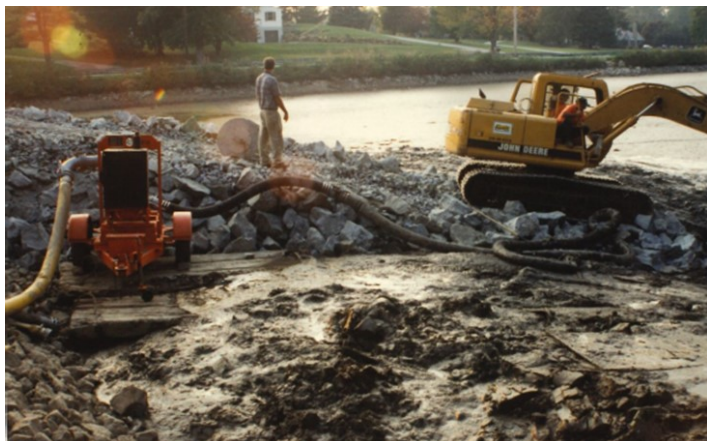
(1997-98) - Supervising installation of trash racks on the Milltown Dam Reservoir outfall pipe
