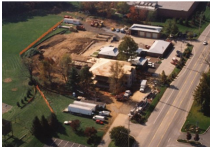
(1992-93) - Township Building construction
