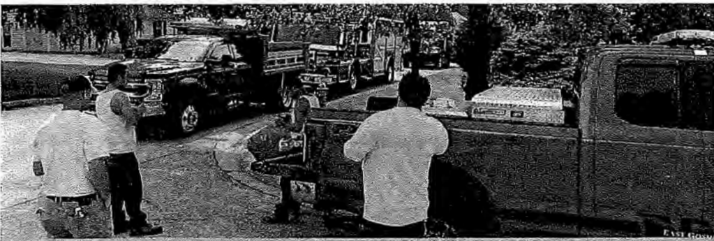
TOP: The public works crews from East Goshen and West Goshen townships in Chester County work together on a road restoration project.
