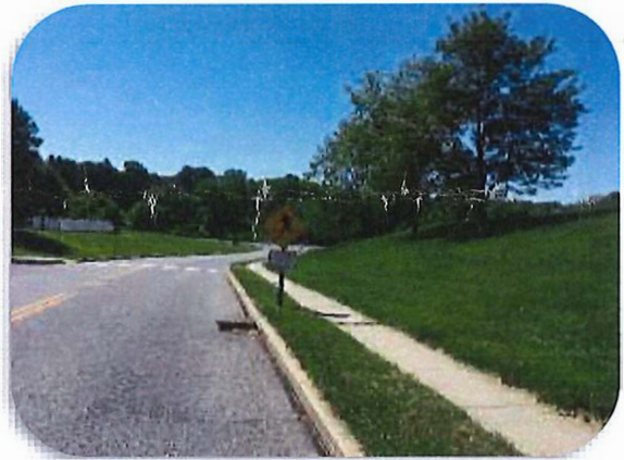
Sidewalk along Skiles Blvd., 2018
