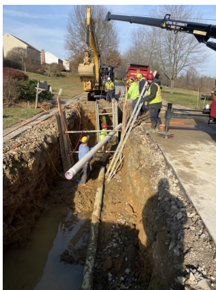
Sewer line repair on Bow Tree Drive
