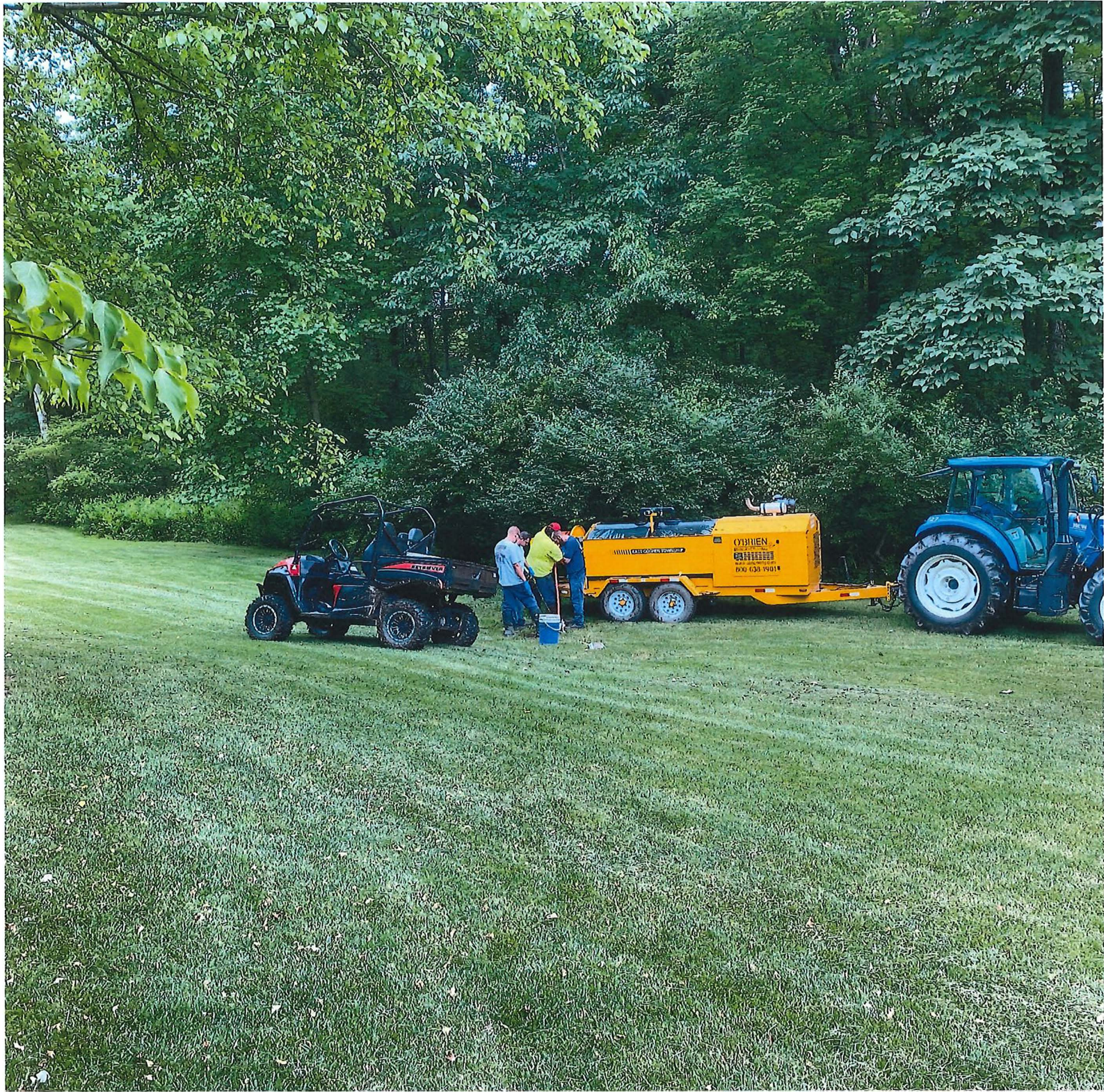
Jetting the Line
