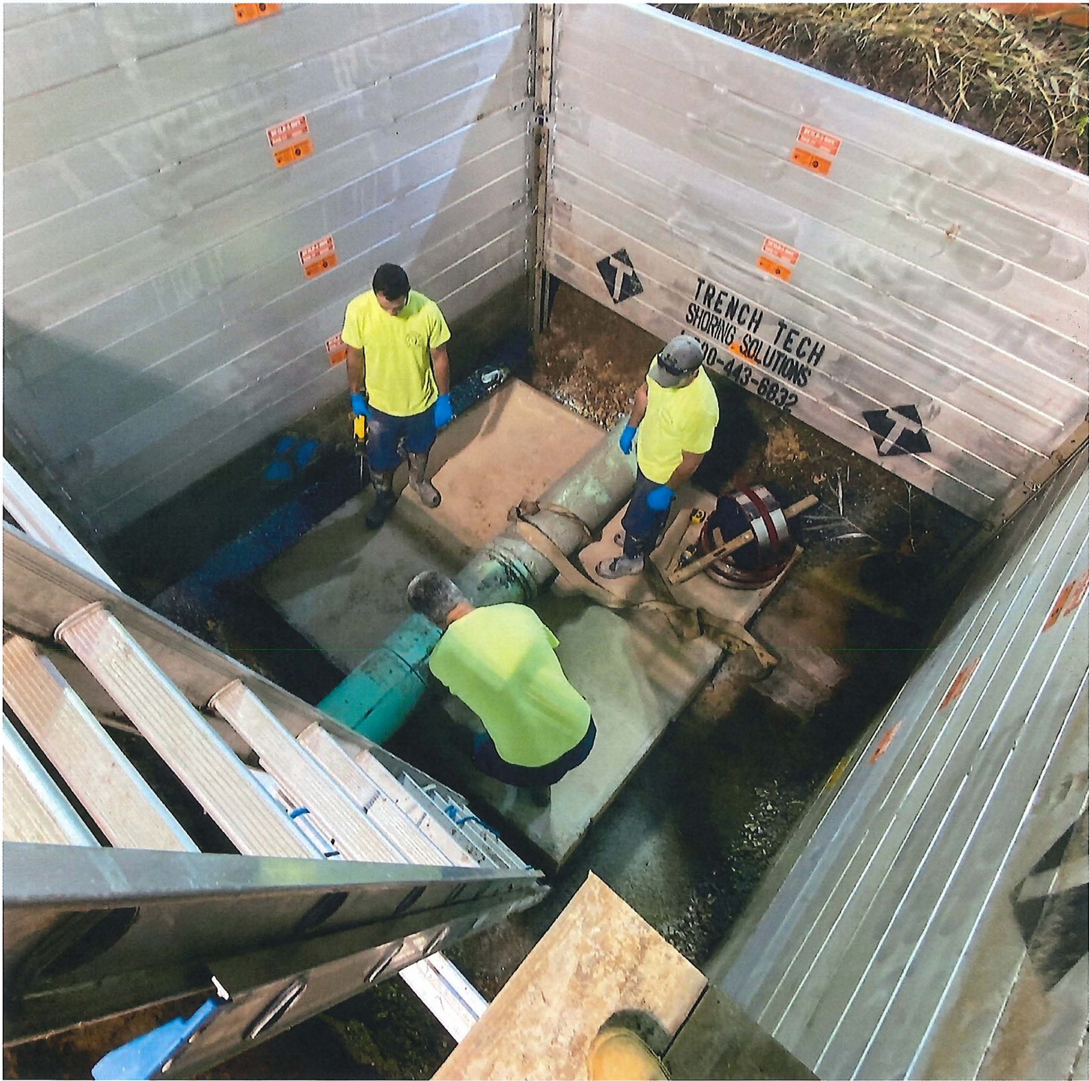
3AM Cut pipe out for Pit
