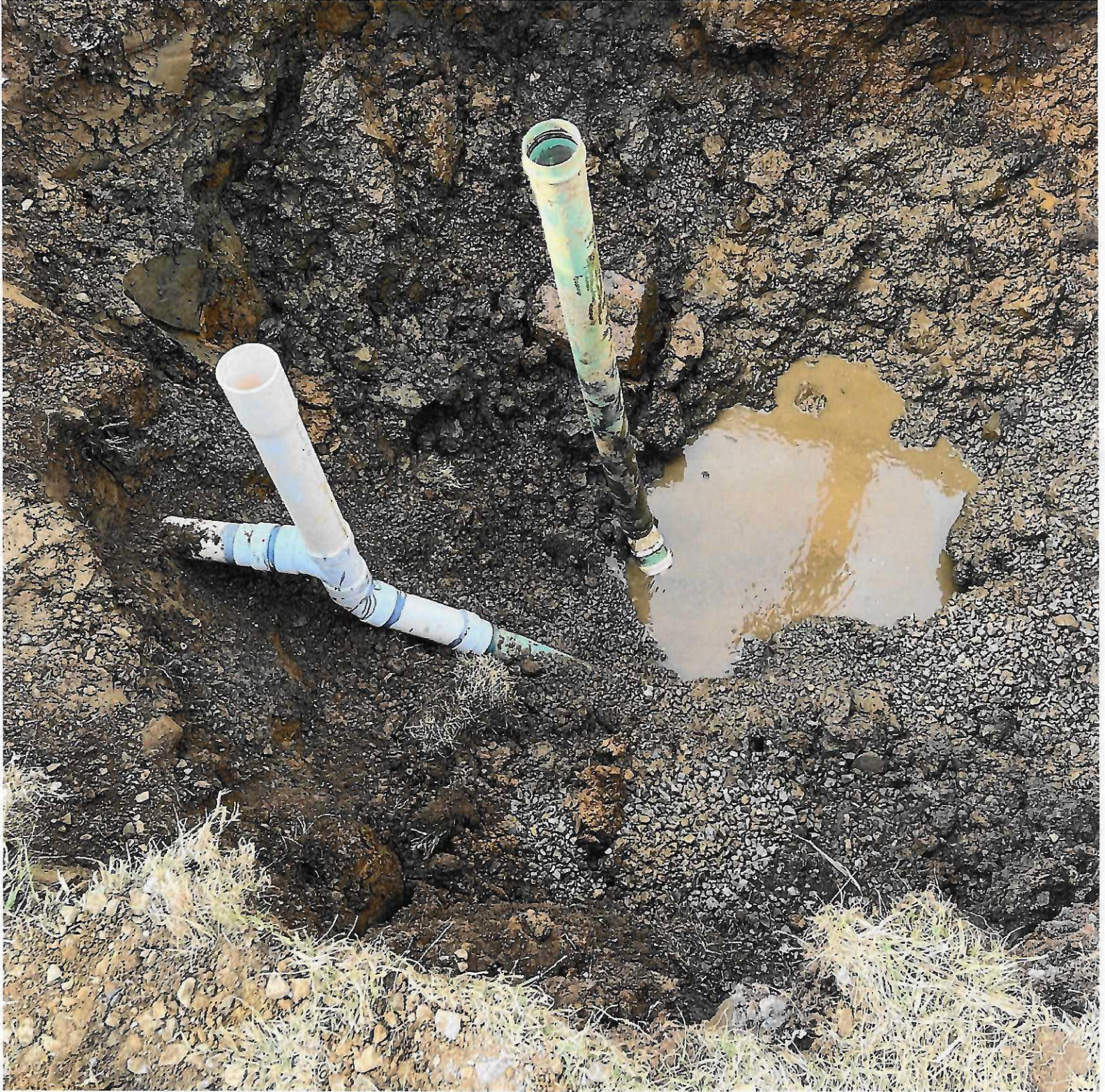
#18 Reservoir Rd. Both lateral's leaking repaired.
