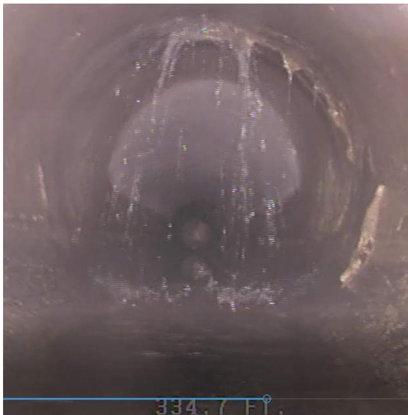
4 - HEAVY RUNNER/CAR WASH AT 20 LF FROM MH C027
