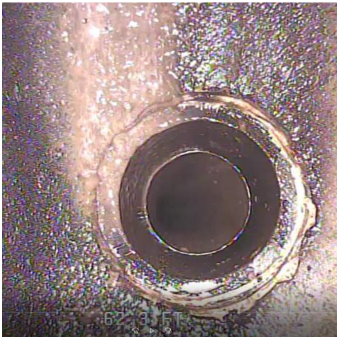
8 - MH C032-C033 – DRIPPER FROM AROUND LATERAL AT 62 FT (Not identified on map since no repair is recommended)
