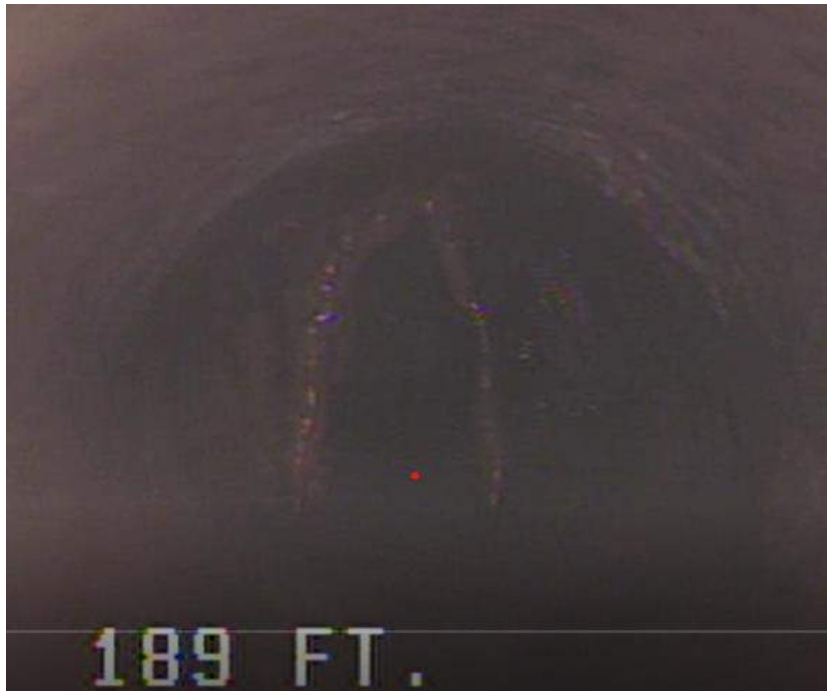
7 – HEAVY RUNNER/CAR WASH IN LATERAL (FROM HOUSE #18 RESERVOIR RD.) @ 189 FT MH C030-C279 (LEAK IS LOCATED SEVERAL FEET WITHIN LATERAL AND PICTURE QUALITY WAS POOR)
