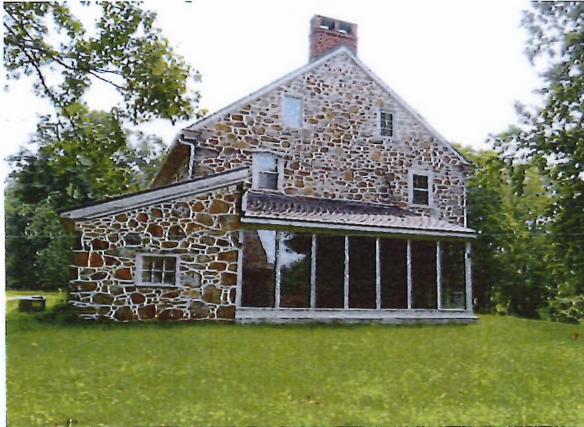
Photograph 07 of 30: Historic Resource #75 – House, showing East elevations of Third Phase (left), Fourth Phase porch (foreground), and First Phase (background), looking Southeast.
