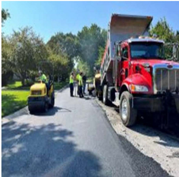
Road resurfacing and maintenance extend the life of our roads.
