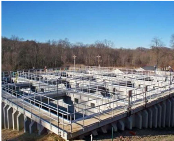
Wastewater treatment infrastructure
