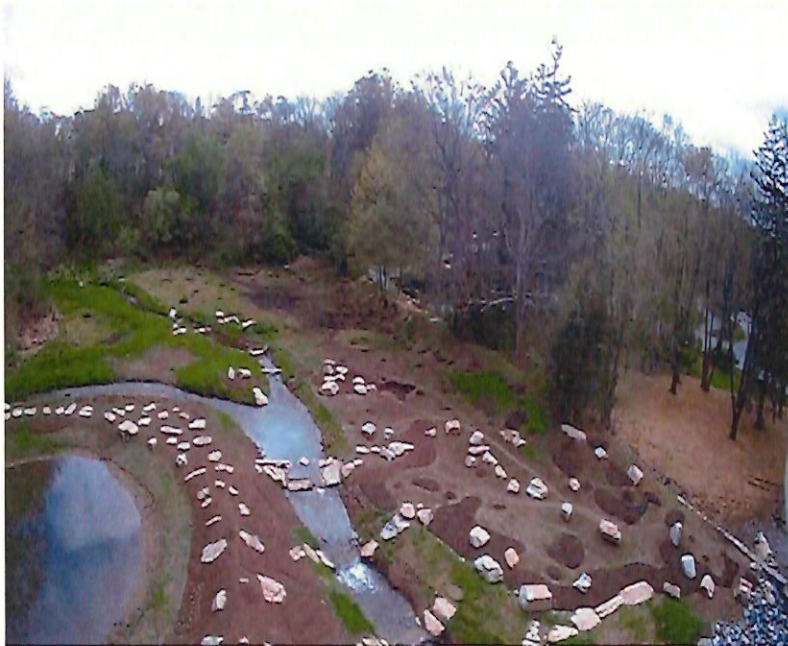
Park and stormwater-related infrastructure
