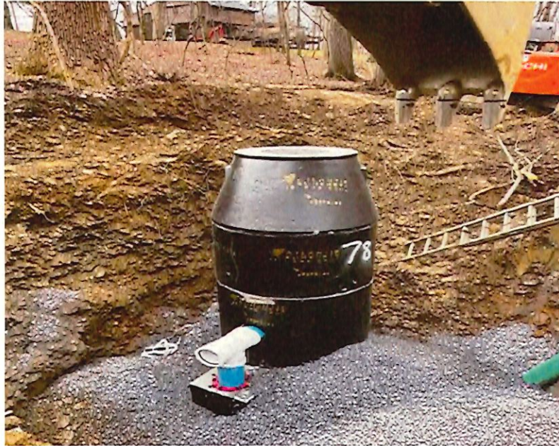
Sewer infrastructure and collection-system improvements
