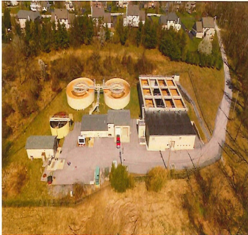
Supporting the infrastructure behind wastewater service
