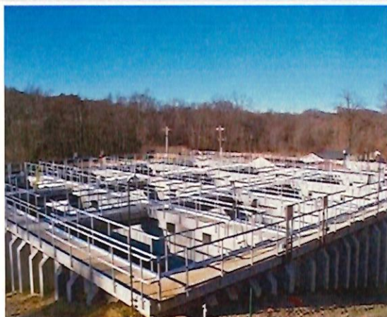
Wastewater treatment infrastructure
